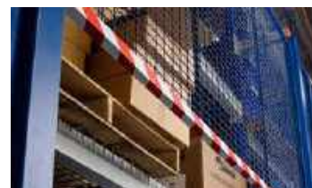
Warn of safety hazards
