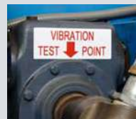
Lean / 5S labeling
